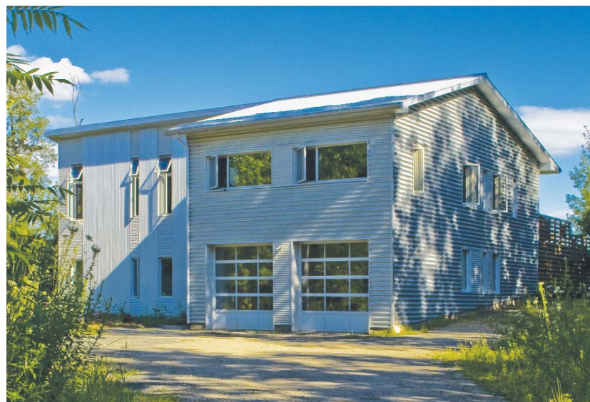
Above The windows on the west, north and east walls are small, to minimize heat loss and capture the more intimate views of the surrounding forest.
