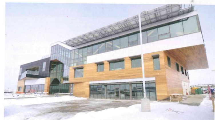
ABOVE Three views of the Mosaic Centre for Conscious Community and Commerce in Edmonton, designed by Manasc Isaac Architects to Passivhaus targets, and supplemented with active solar components.
